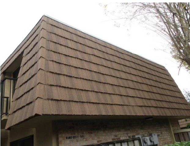
MANSARD WALLS REPLACED 2018
