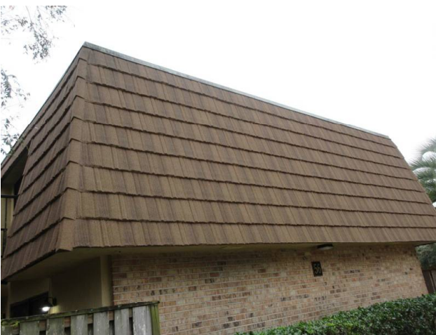
MANSARD WALLS REPLACED 2018
