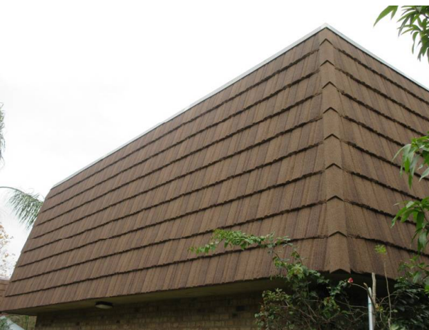
MANSARD WALLS REPLACED 2018
