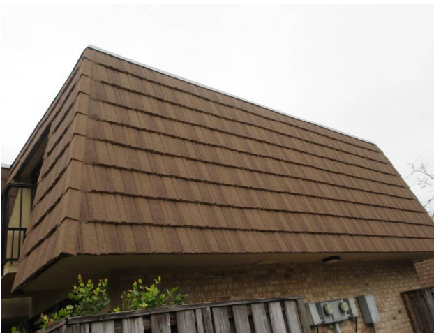
MANSARD WALLS REPLACED 2018
