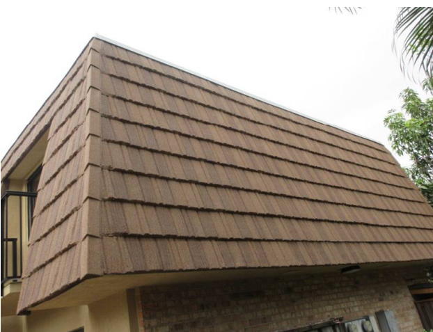
MANSARD WALLS REPLACED 2018
