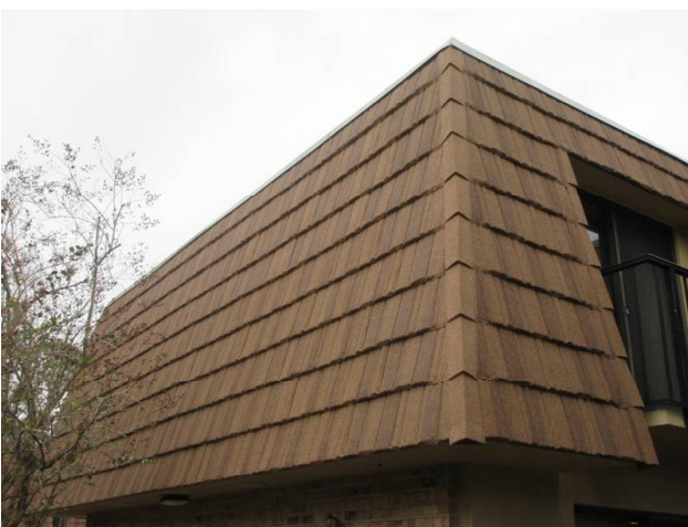
MANSARD WALLS REPLACED 2018
