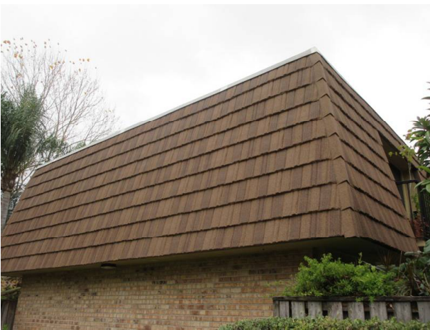
MANSARD WALLS REPLACED 2018
