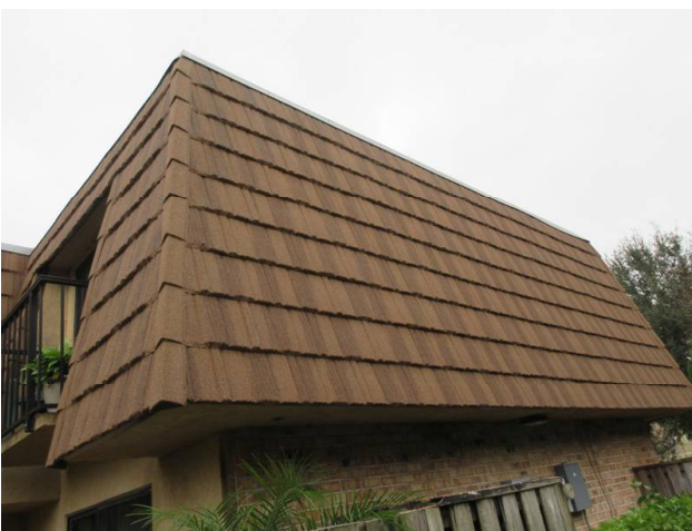
MANSARD WALLS REPLACED 2018
