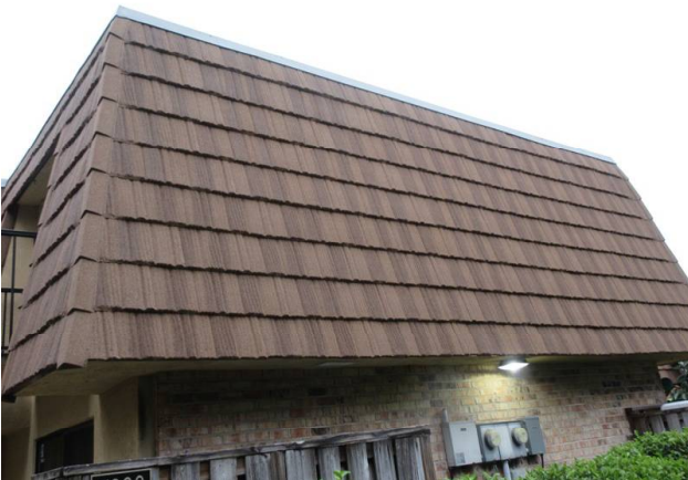
MANSARD WALLS REPLACED 2018
