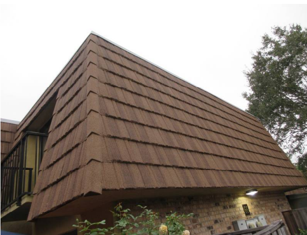
MANSARD WALLS REPLACED 2018
