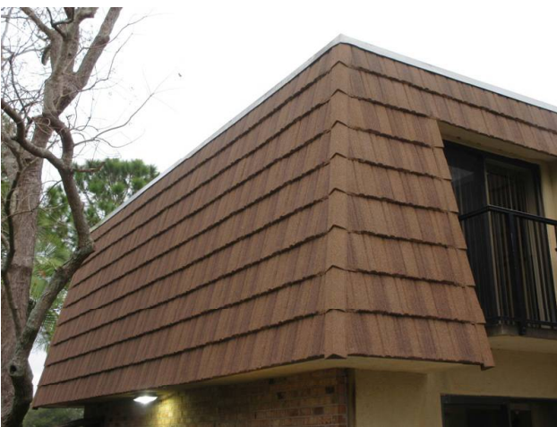
MANSARD WALLS REPLACED 2018
