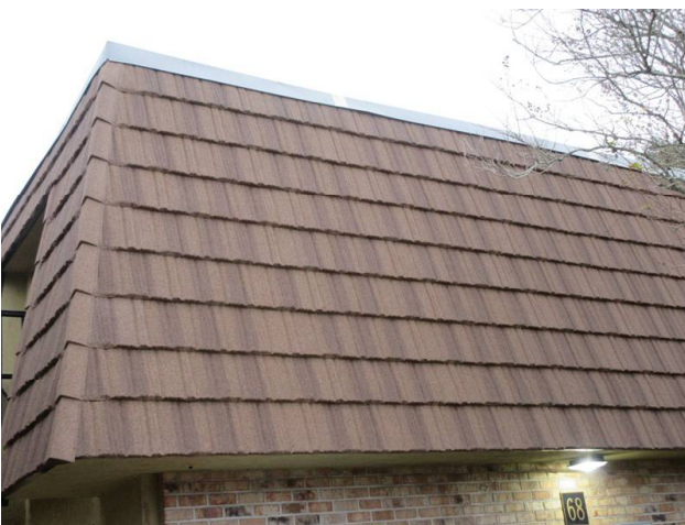
MANSARD WALLS REPLACED 2018
