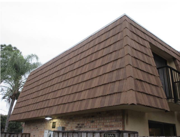
MANSARD WALLS REPLACED 2018
