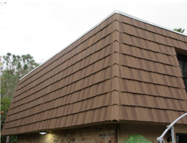
MANSARD WALLS REPLACED 2018
