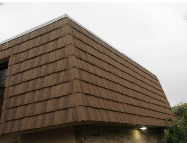
MANSARD WALLS REPLACED 2018
