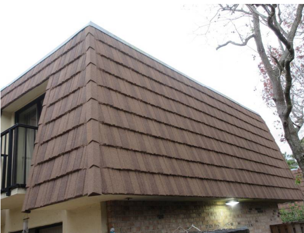
MANSARD WALLS REPLACED 2018
