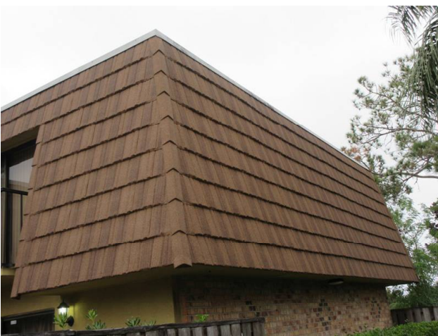
MANSARD WALLS REPLACED 2018
