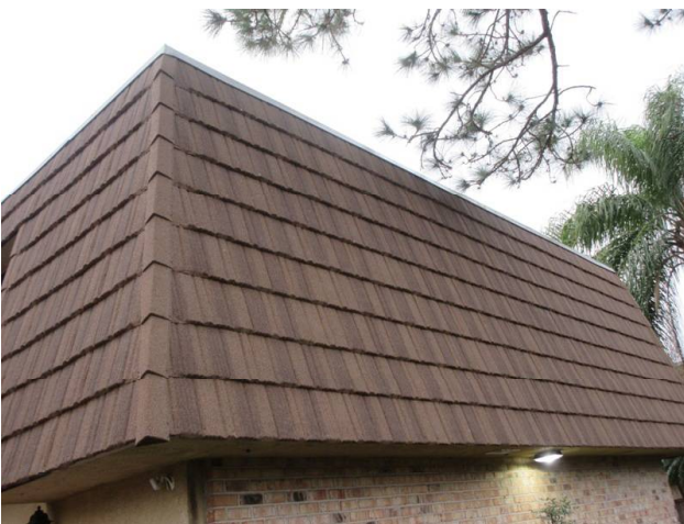
MANSARD WALLS REPLACED 2018
