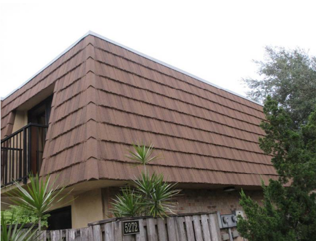
MANSARD WALLS REPLACED 2018
