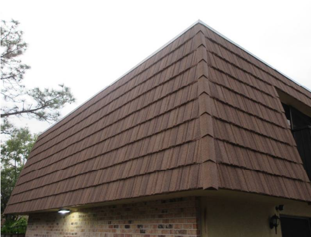
MANSARD WALLS REPLACED 2018
