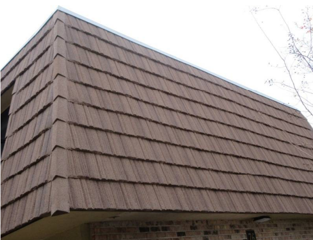
MANSARD WALLS REPLACED 2018
