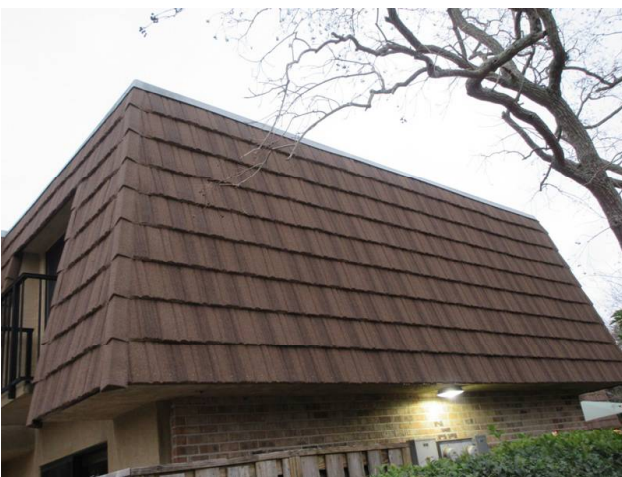
MANSARD WALLS REPLACED 2018
