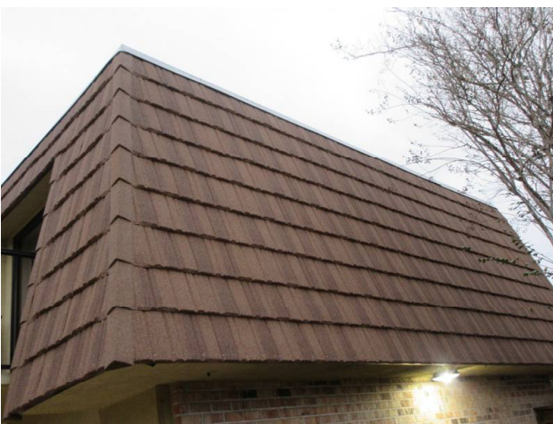
MANSARD WALLS REPLACED 2018
