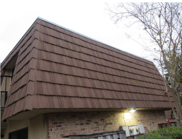
MANSARD WALLS REPLACED 2018
