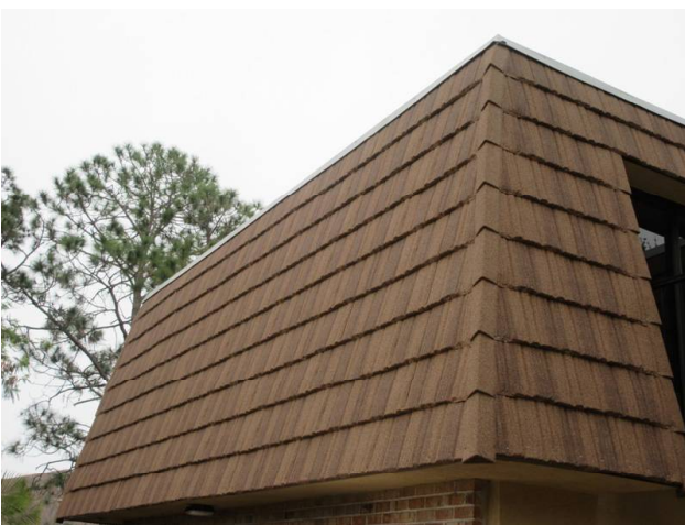
MANSARD WALLS REPLACED 2018
