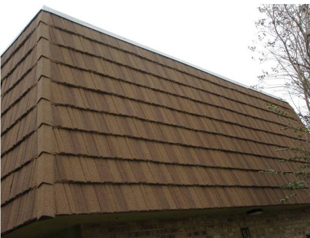
MANSARD WALLS REPLACED 2018
