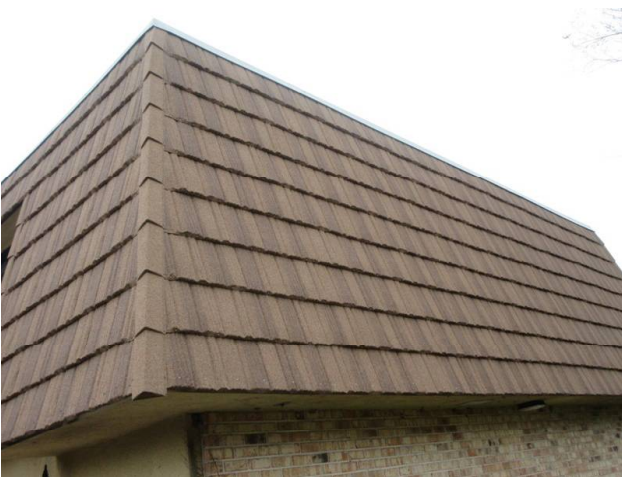
MANSARD WALLS REPLACED 2018
