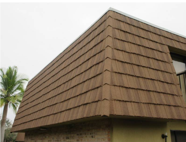
MANSARD WALLS REPLACED 2018
