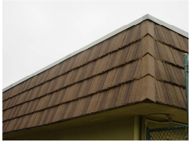
MANSARD WALLS REPLACED 2018
