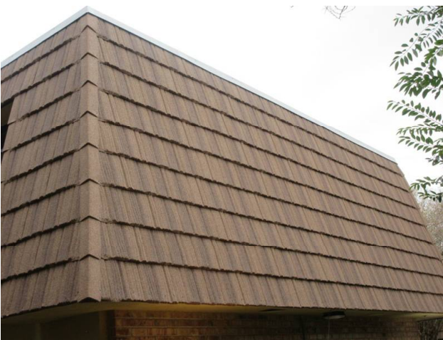
MANSARD WALLS REPLACED 2018
