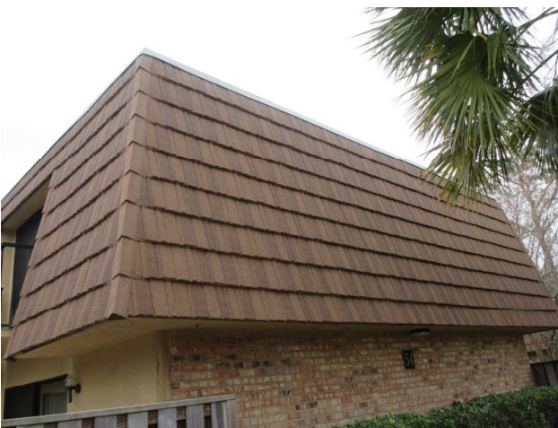
MANSARD WALLS REPLACED 2018
