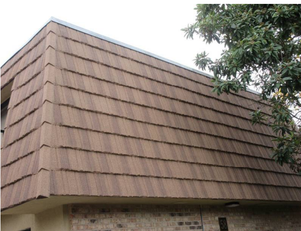
MANSARD WALLS REPLACED 2018
