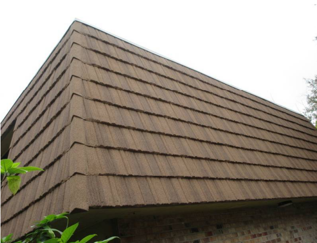
MANSARD WALLS REPLACED 2018
