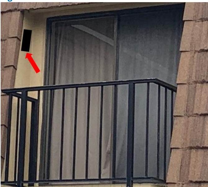
Figure 4.A - The contractor will need to remove a small portion (1'x1') in 2 areas of the exterior wall of the mansard styled siding as shown with the red arrows. A hole in the soffit above the balcony is optional if it becomes difficult to run the refrigerant lines through the interior portion of the overhang (as shown with the red arrows) .
