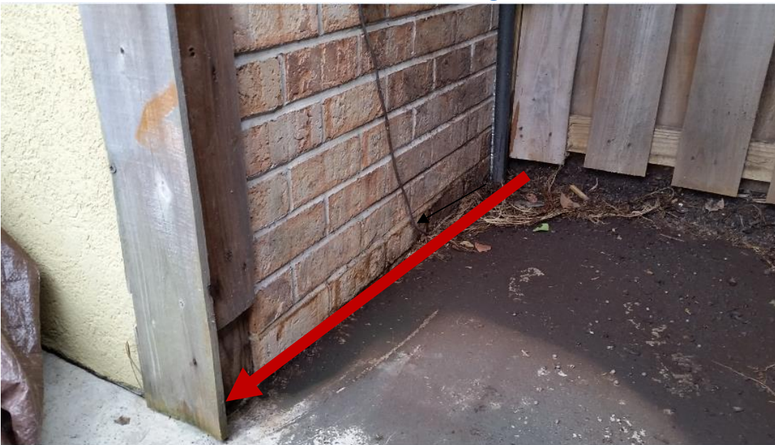
Figure 2 – The refrigerant lines will enter the storage area at ground level and run to the receiving post of the storage gate (as shown with the red arrow).
