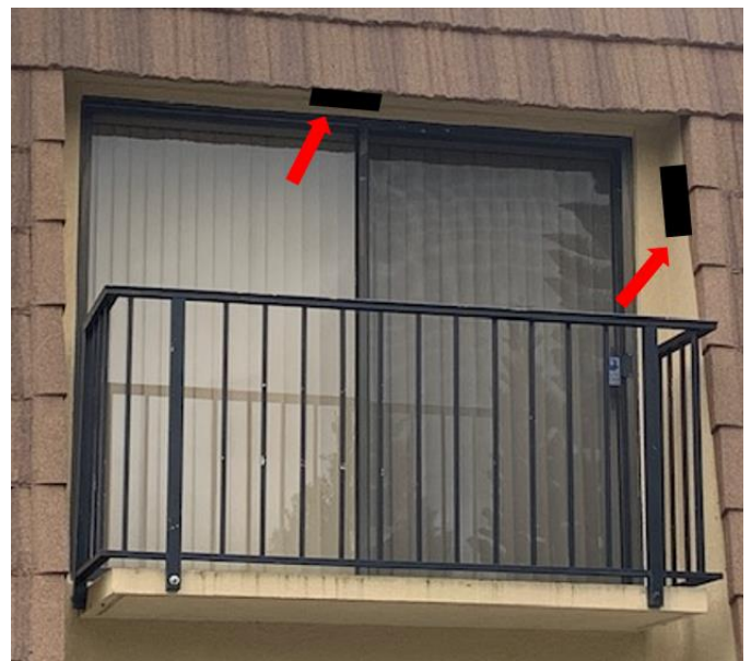
Figure 4.A - The contractor will need to remove a small portion (1'x1') in 2 areas of the exterior wall of the mansard styled siding as shown with the red arrows. A hole in the soffit above the balcony is optional if it becomes difficult to run the refrigerant lines through the interior portion of the overhang (as shown with the red arrows) .
