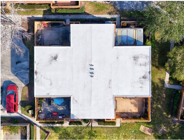
ROOF - CONCRETE WITH TPO COVERING
