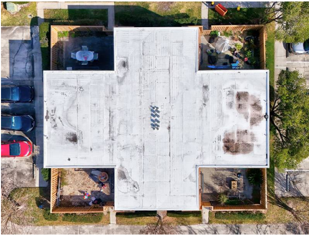
ROOF - CONCRETE WITH TPO COVERING
