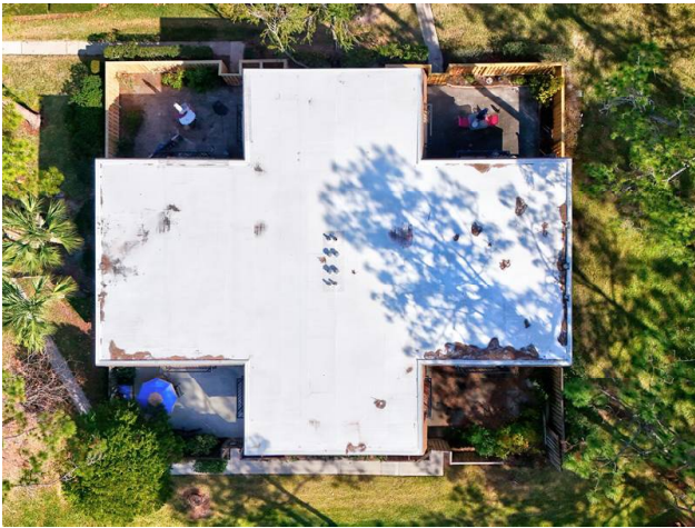
ROOF - CONCRETE WITH TPO COVERING
