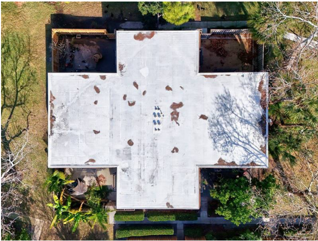
ROOF - CONCRETE WITH TPO COVERING
