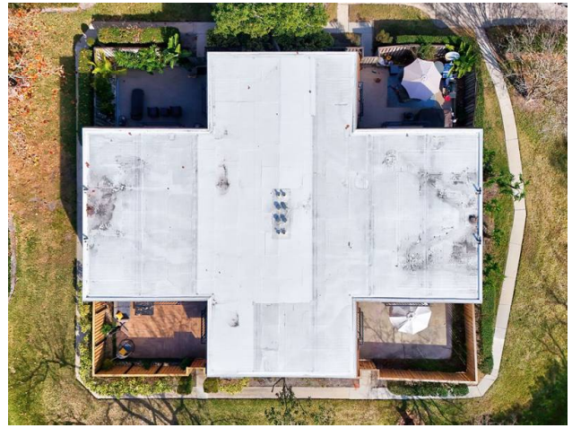
ROOF - CONCRETE WITH TPO COVERING
