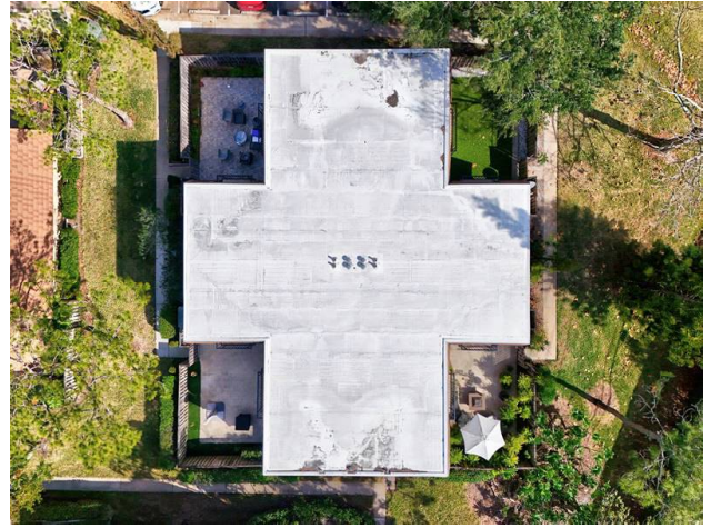
ROOF - CONCRETE WITH TPO COVERING
